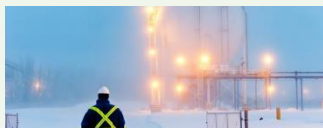
Electrolyzer in Quebec
